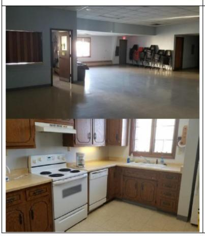
Kitchen counters and the serving counter are 3' high not at the ADA standard 2'-10". Stove exhaust needs to be vented to the exterior. The kitchen is more residential style in nature and in need of remodel. Commercial ventilation should be installed.
