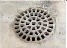
Floor drains frequently don't drain because of too much sediment coming off of trucks. Many hours are spent by staff cleaning these. Repairs should be made to these drain locations.
